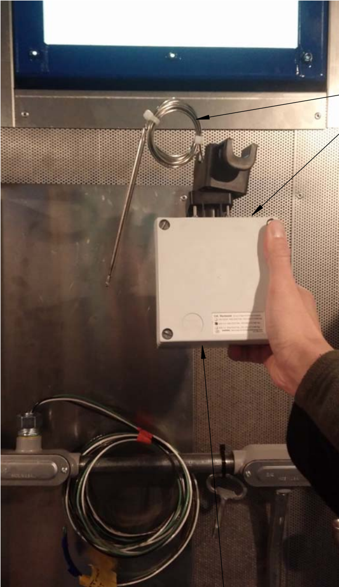
MS-E4X-1-H - HEAT TRACE THERMOSTAT - SHOWN IN APPROXIMATE LOCATION
