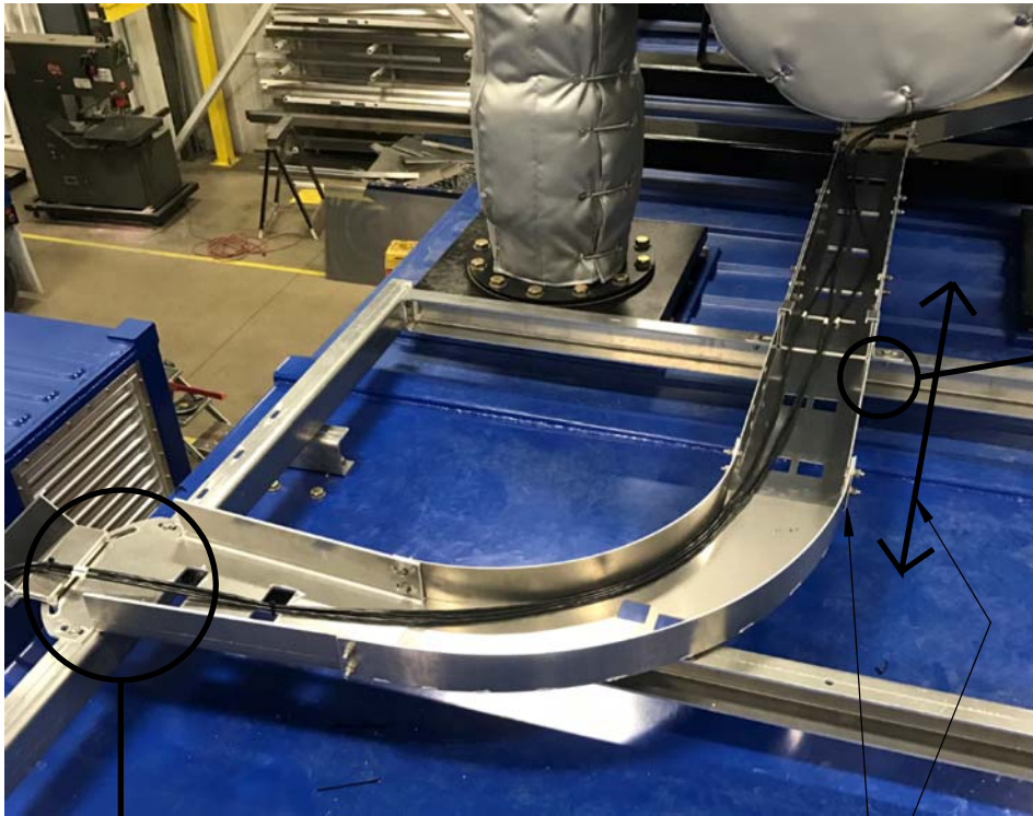
ADJUST LENGTH OF CABLE TRAY AS NECESSARY
