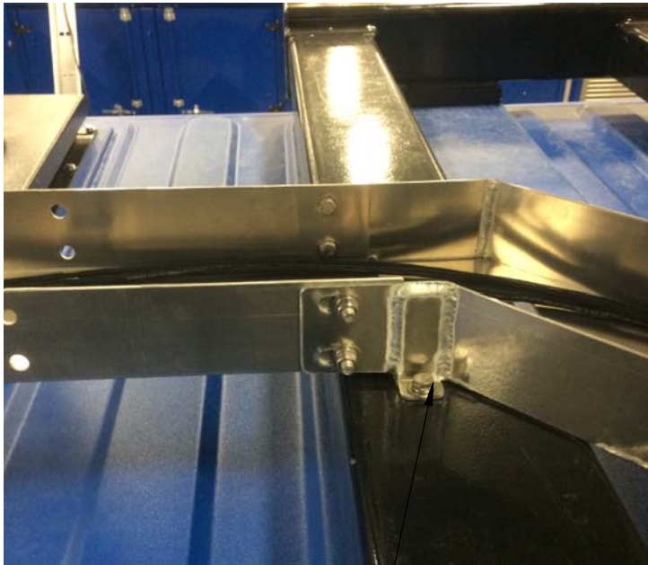
BOLT LOOSE CABLE TRAY PIECE TO PRE-INSTALLED TRAY PIECE ON SCR SKID
